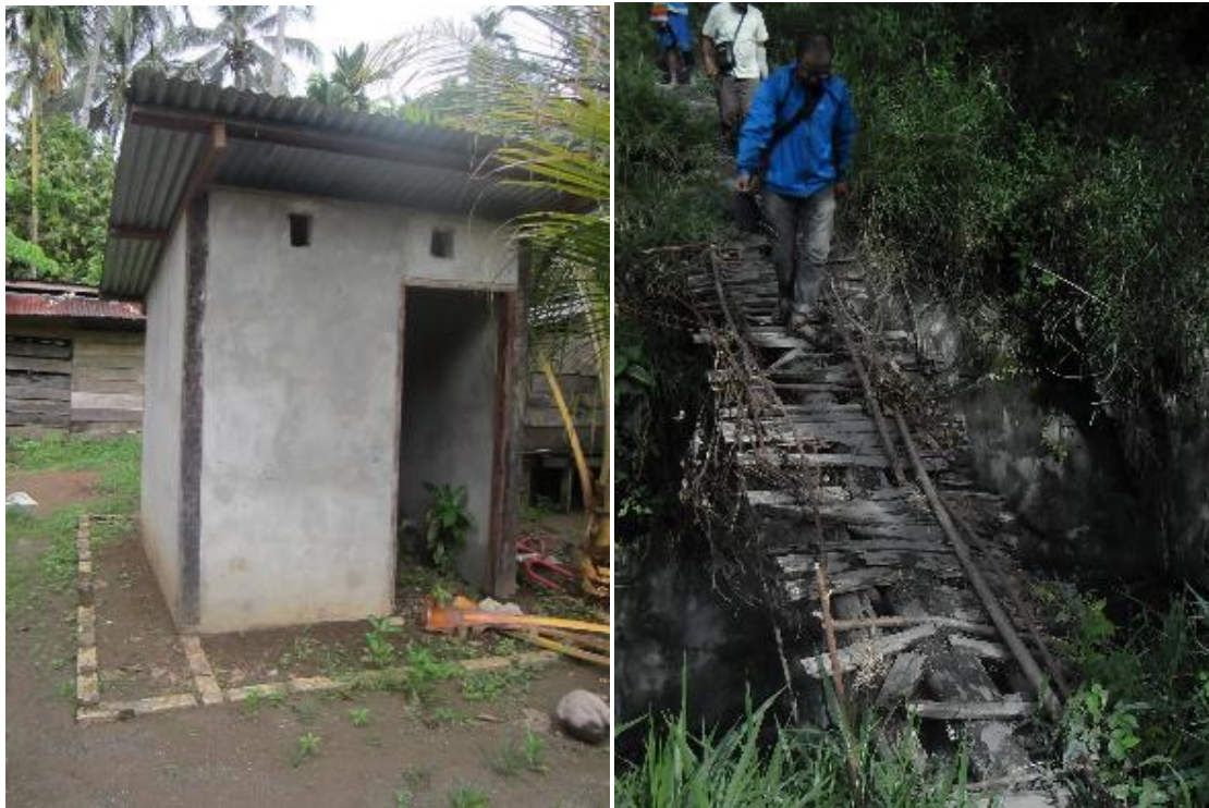
Latrine (2013) in Sawesuma, Unurum Guay, Jayapura
