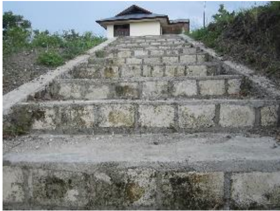
Figure 8 Concrete staircase, Ifar Besar, Sentani.
